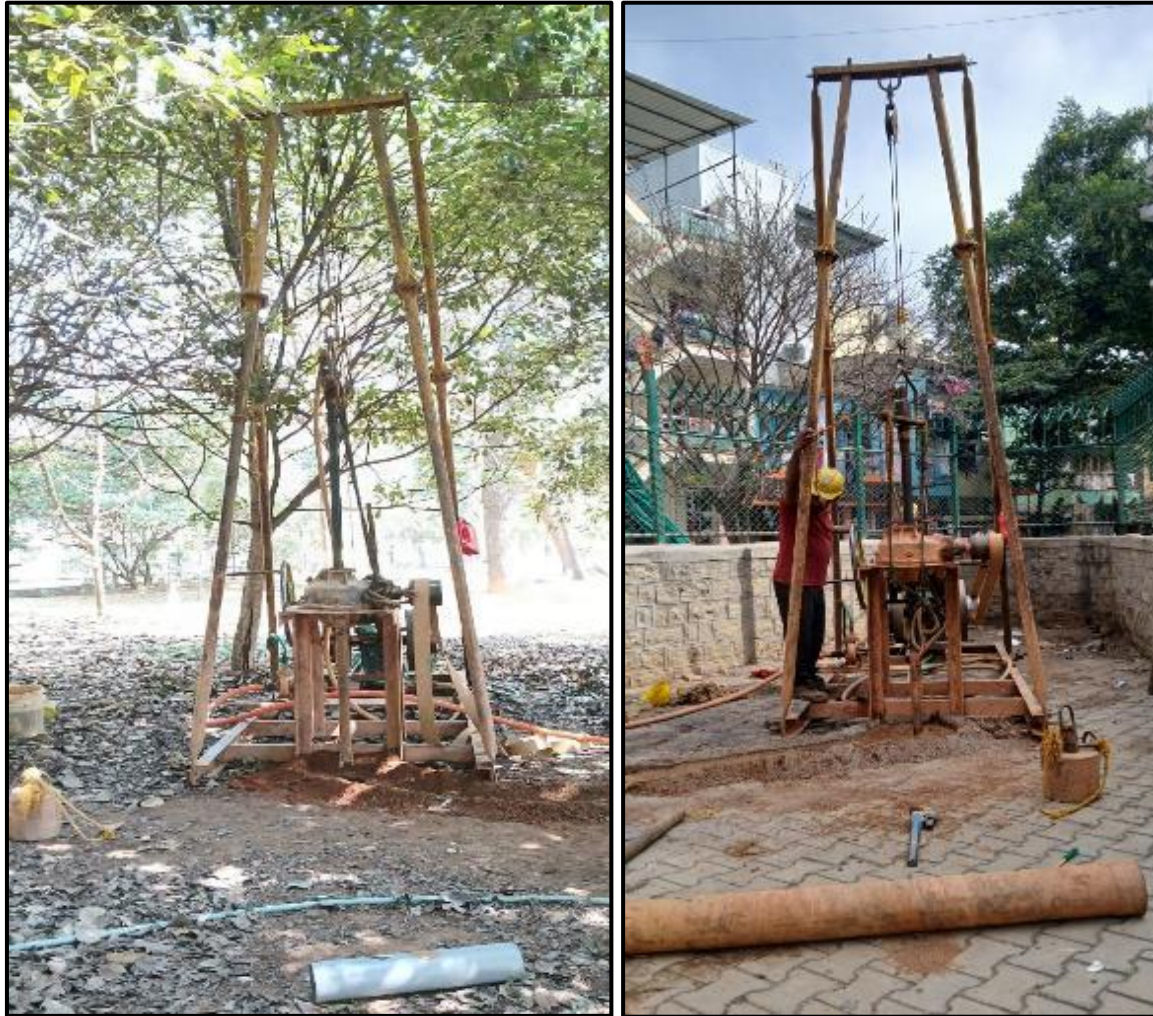
Figure 52: Ongoing Borehole along proposed tunnel alignment
